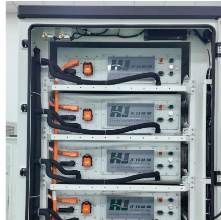
Sunny Inspire , PV Solar Panel , Battery storage
