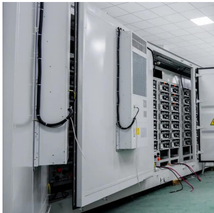
5G Base Station Power Supply with Battery & DC Distribution
