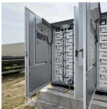
**60kWh Air-Cooling Battery Energy Storage System ,**
